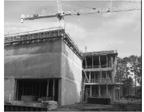
Construction of new facility entrance
